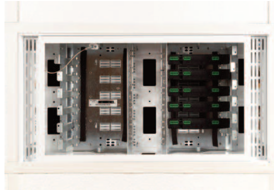
FSR partnered with Platformatics to secure lighting nodes in the ceiling boxes for zone cabling architecture.
